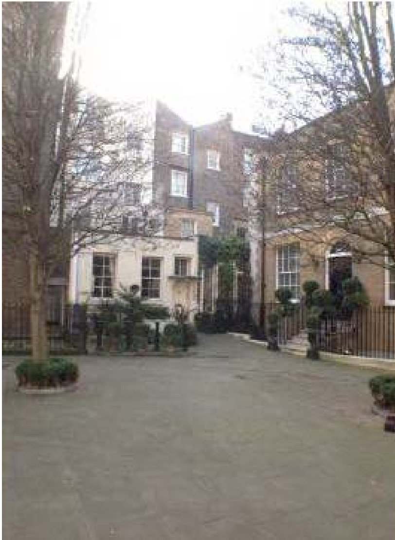
View of the rear of application property (existing brick extension) from Wyndham Place
